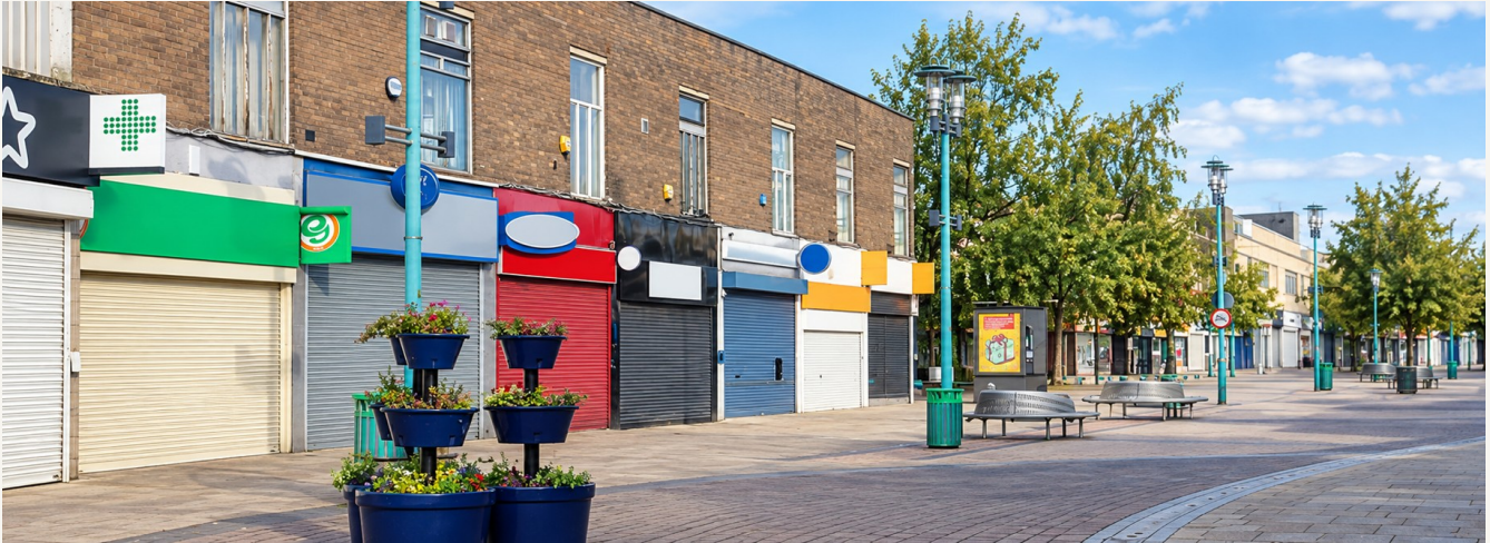
Huyton town centre · Cavendish Walk, at the heart of the borough's largest town-centre scheme.
