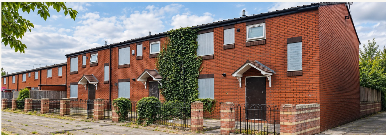
Collyhurst · Existing streets within the Victoria North area.
