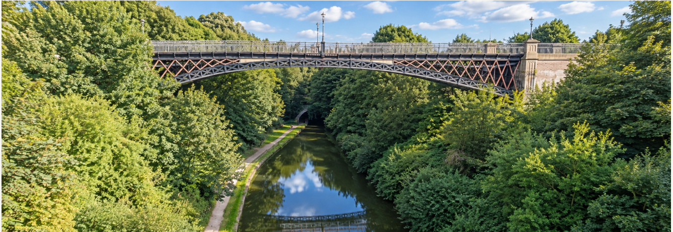
Galton Bridge · The Birmingham Canal Old Line at Smethwick.
