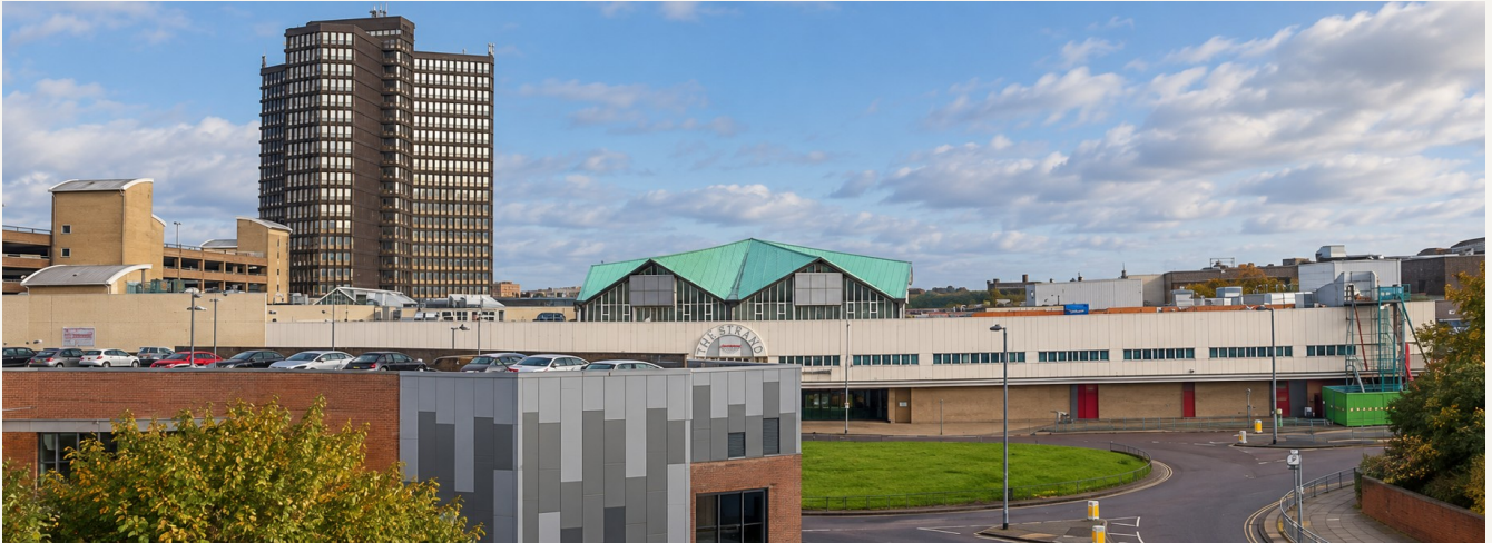
Bootle Strand · Phase 1 under construction, completing spring 2027.
