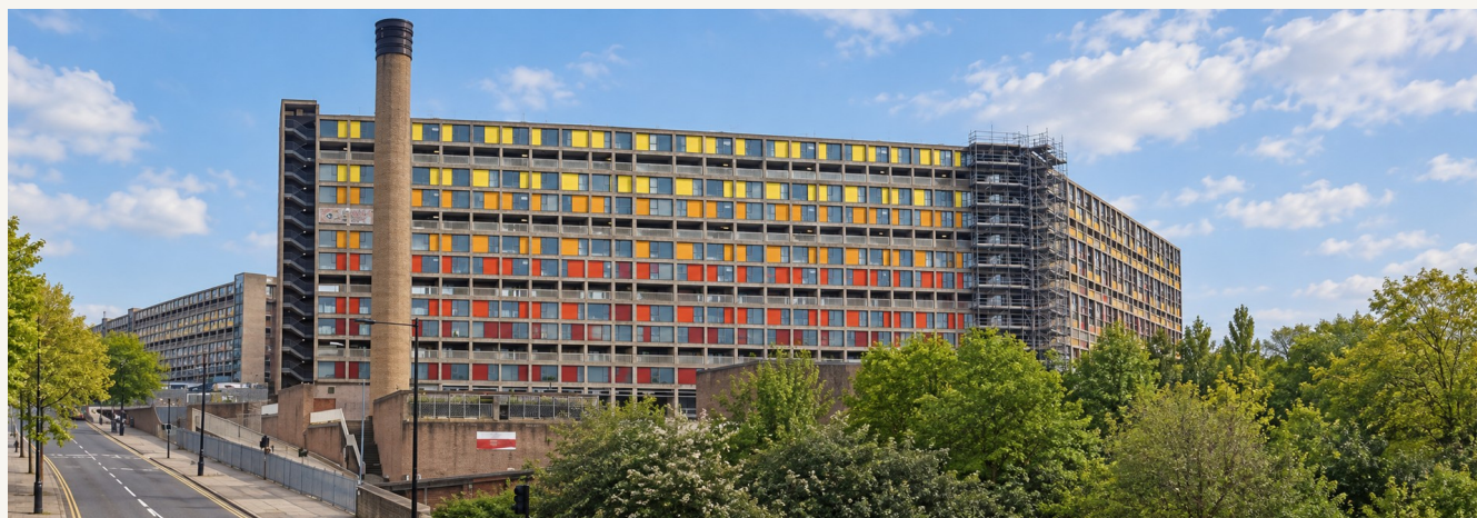
Park Hill · The renovated flats above the station.
