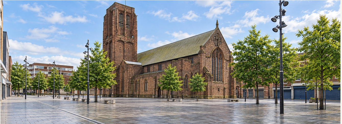
St Helens town centre · Phase 1A is on site within the wider c.£100m ECF masterplan.
