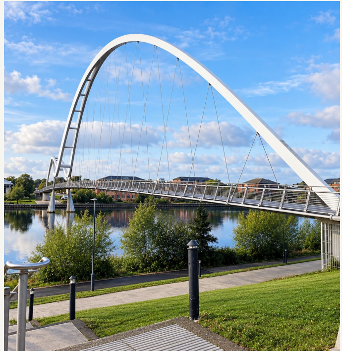
Infinity Bridge, Stockton
