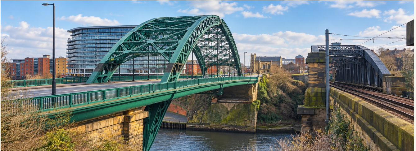
River Wear · Wearmouth Bridge and the railway bridge.
