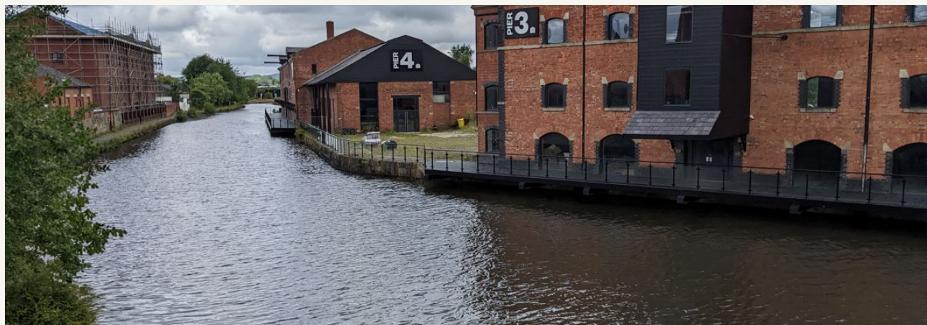
Wigan Pier · Former industrial buildings beside the Leeds and Liverpool Canal.
