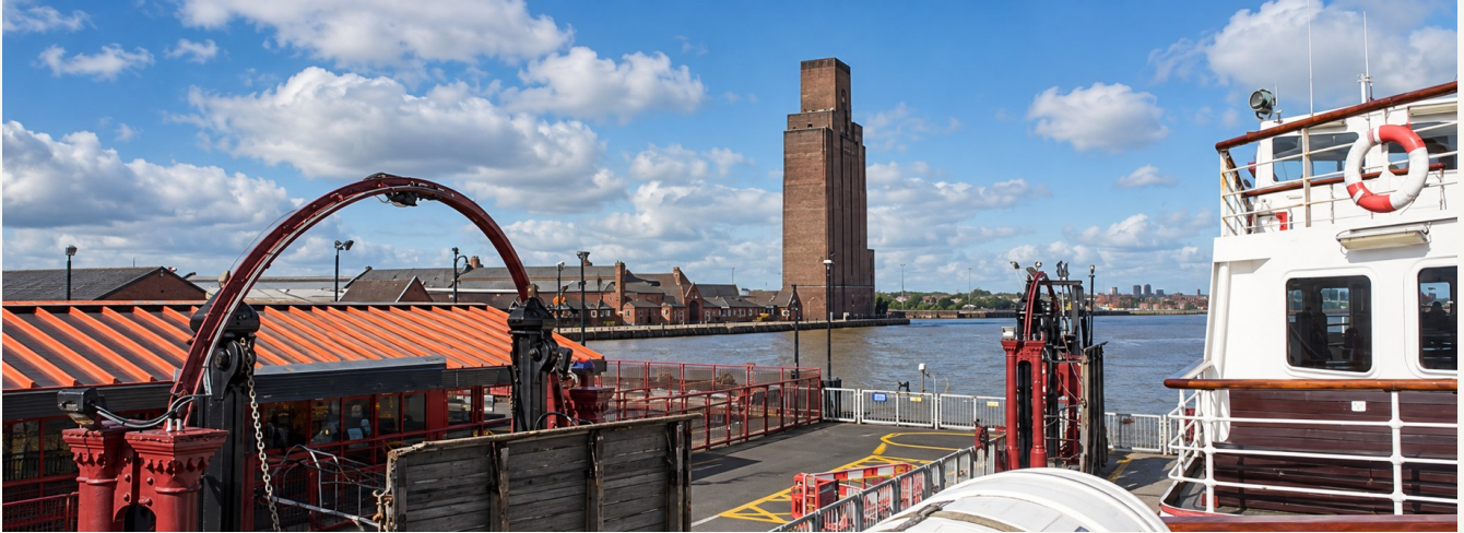
Woodside · The Birkenhead waterfront at the ferry terminal, south of Wirral Waters.
